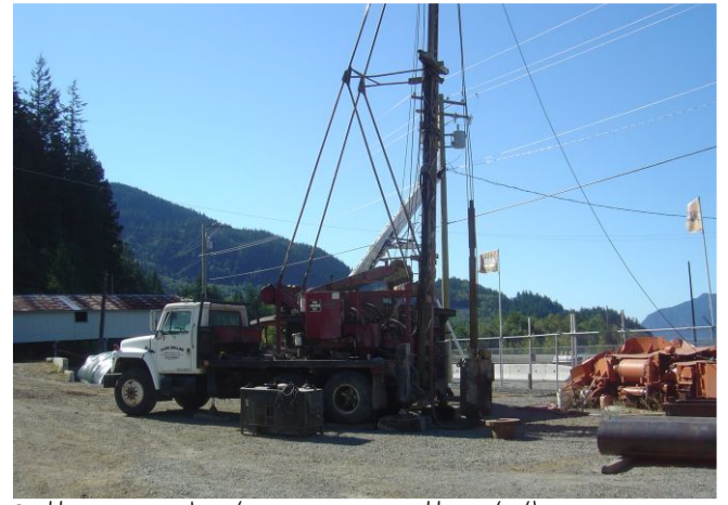
Drilling groundwater pumping wells at the Museum
