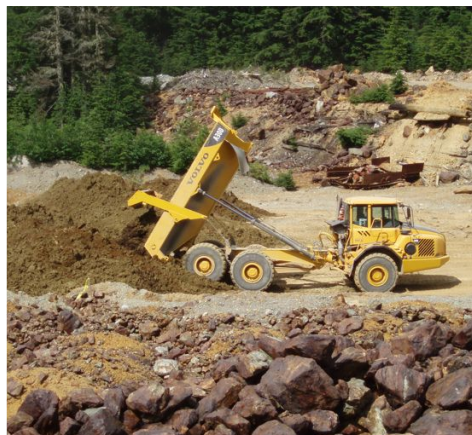
Dumping sludge in the Jane Basin
