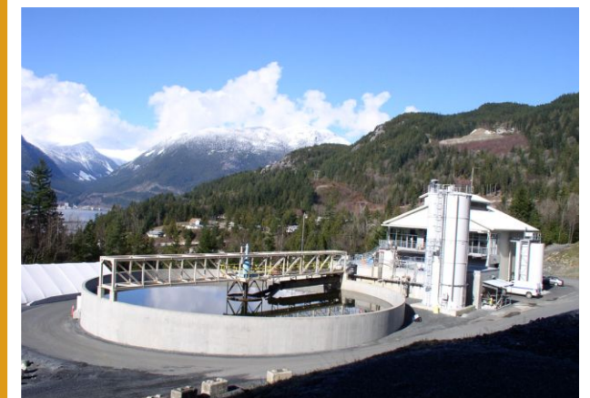
EPCOR Water Treatment Plant
