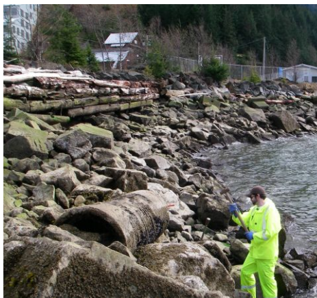
installing a piezometer, 2008
