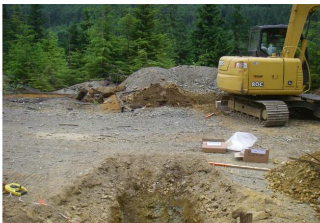
Test pitting near the 2200 Level portal in 2008
